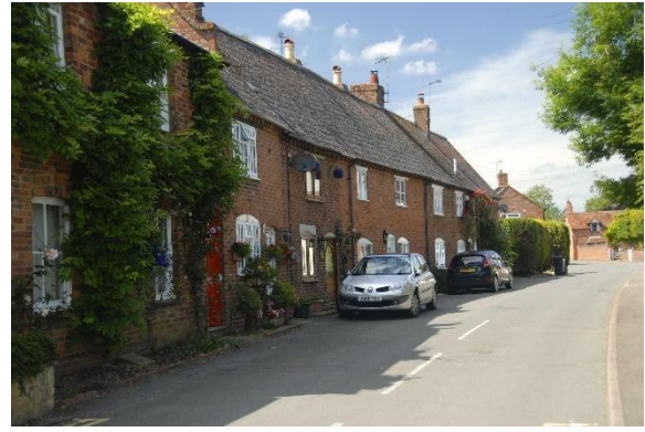
Lower Street Cottages looking north
